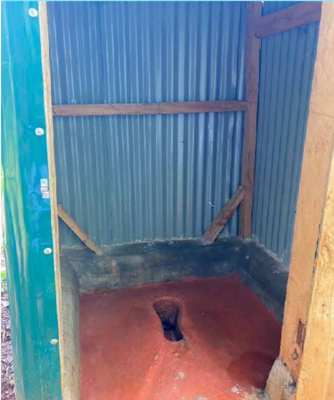
Pit latrine with slab that meets our standard.
