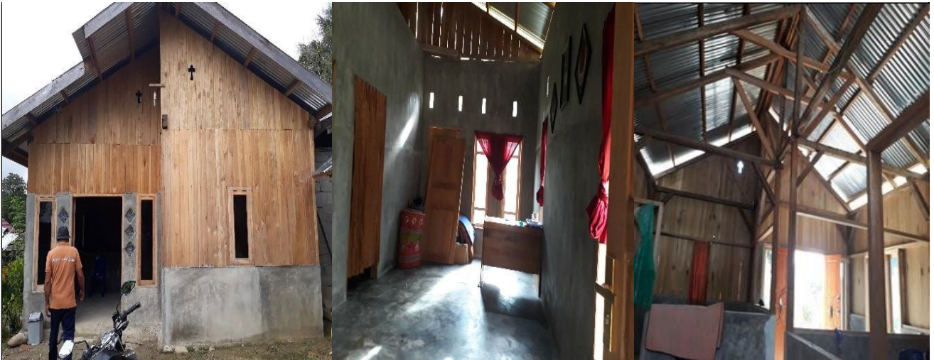
Figure 14 A newly constructed house in Kulawi
